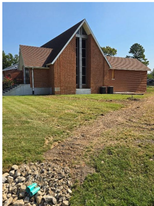
Trinity Lutheran Church Addition
